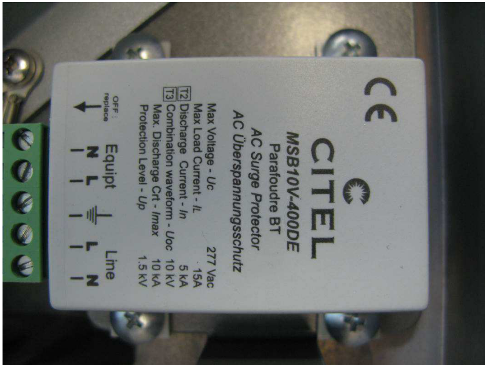
Photo 5) VFL540 S70.BEAM 48 LED – 108W 4000°K SurgeProtector
